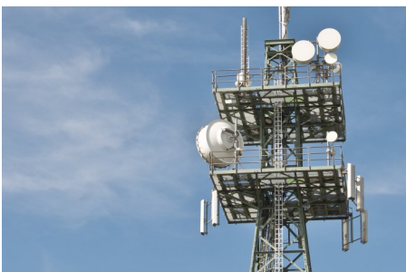
Indonesia's telecommunication tower
